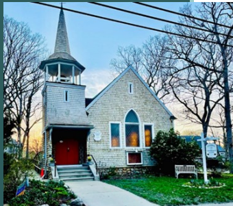
Freshly power washed Chapel
